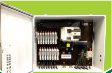
String Combiner Box
